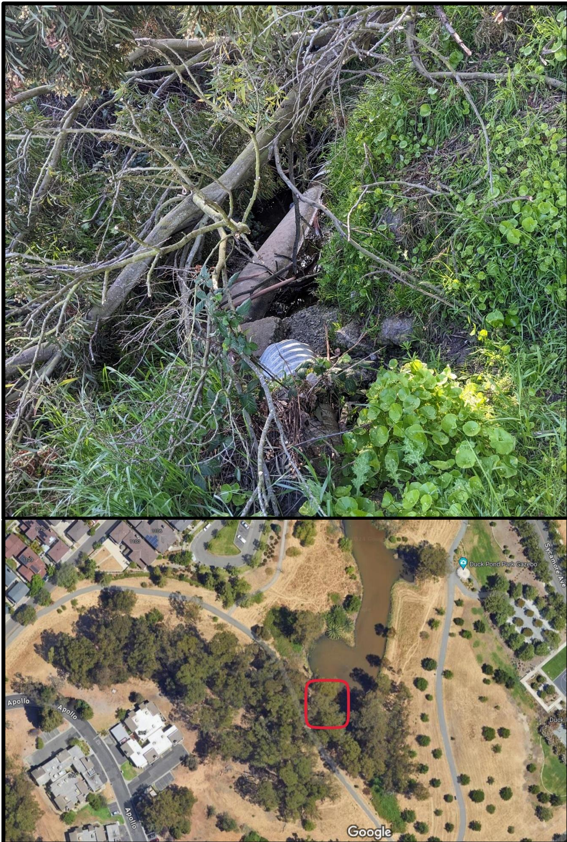
Figure 2 – Exposed Force Main Photograph and Location
